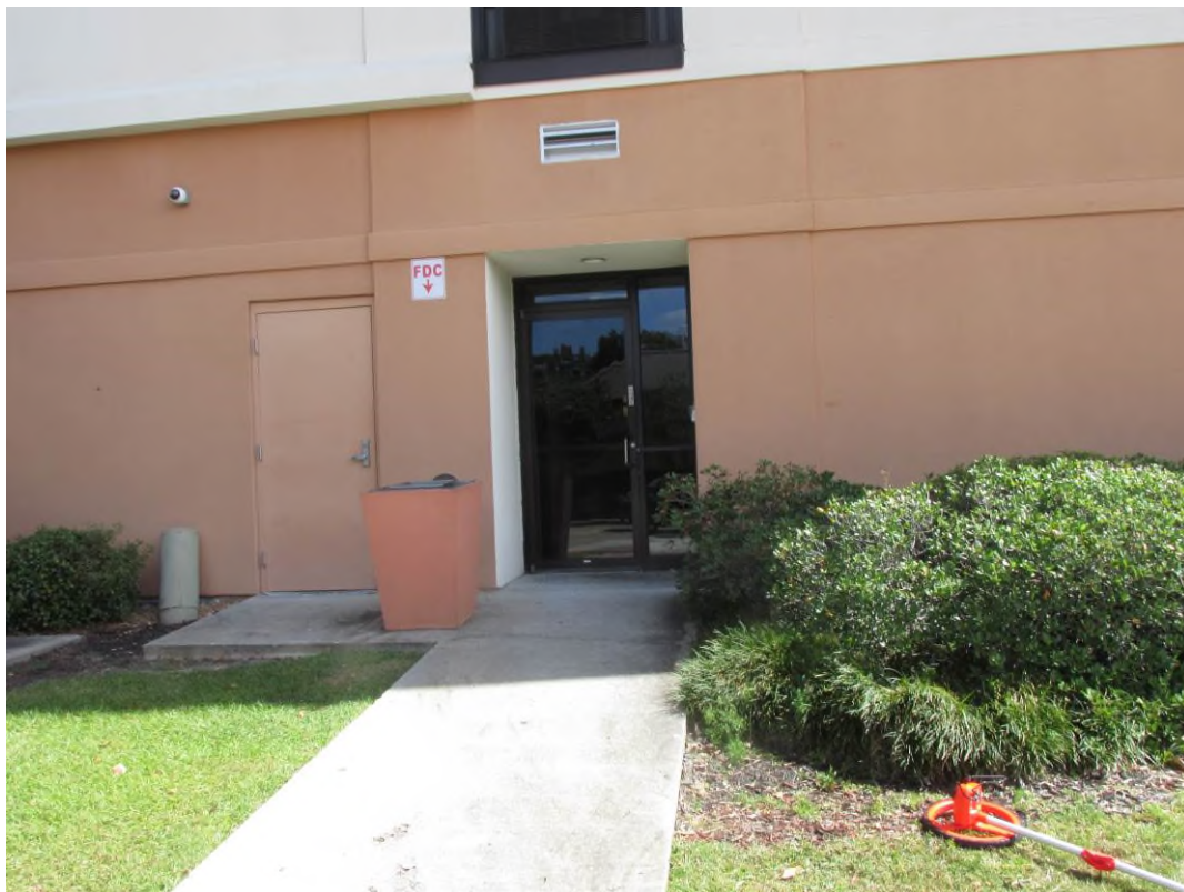
Hyatt side door begins at a distance of 97 feet including 11 feet for electric vault
