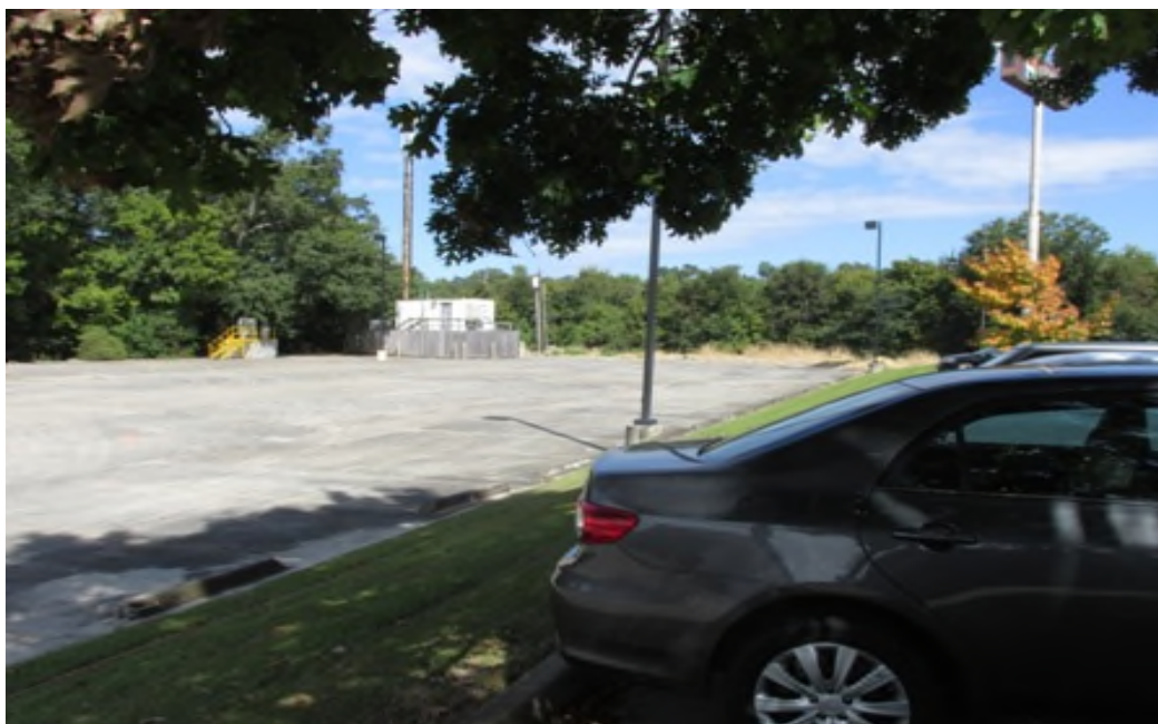
Cell tower and parking below Hyatt grade on rear lot of Ralph & Kacoo's to be separated by Dijon Dr. from restaurant
