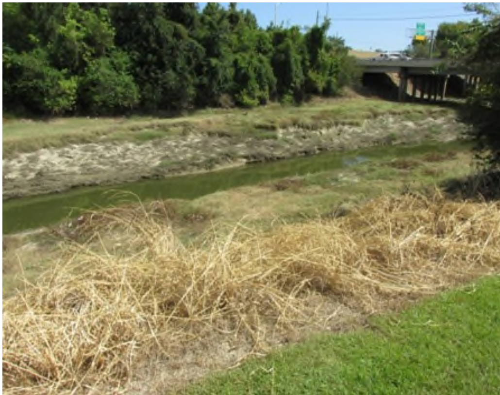
East side steep drainage ditch area limits any new parking access road
