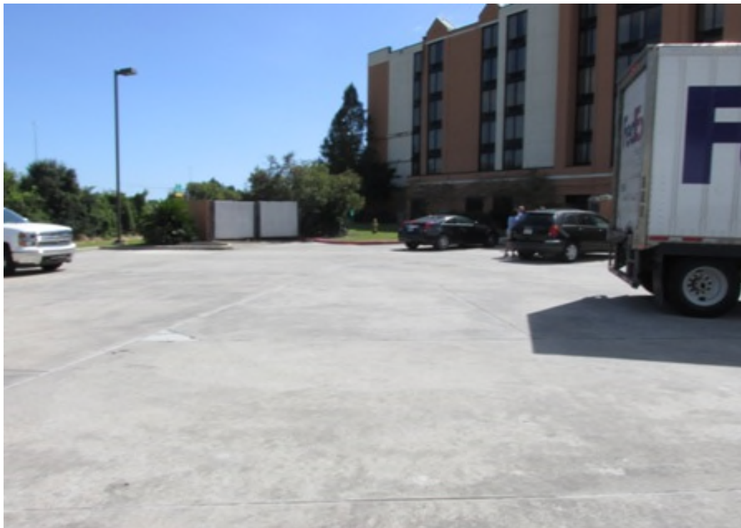
Rear parking access from east is mostly blocked by trash and dumpster and outdoor pool areas, fire lane and fire hydrant
