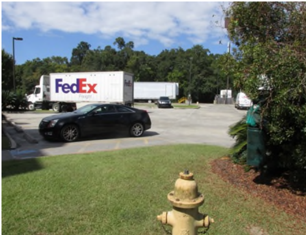
Location for narrow new access road would require relocation of fire hydrant
