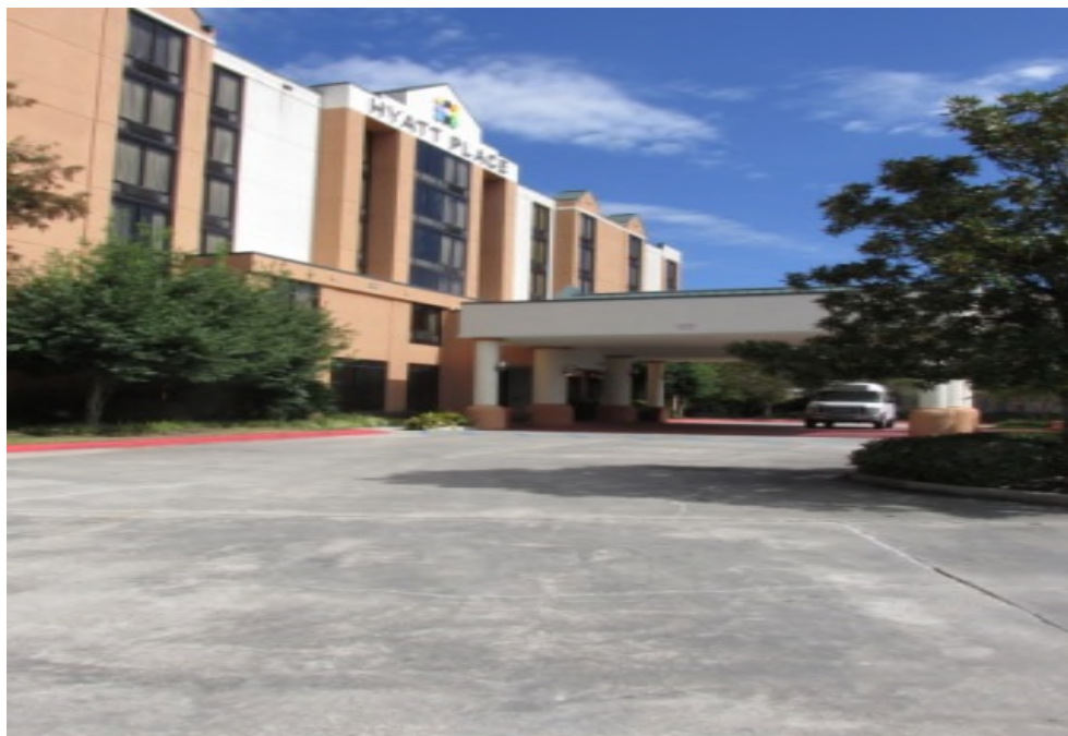
Front view from entry of quiet Hyatt Place site
