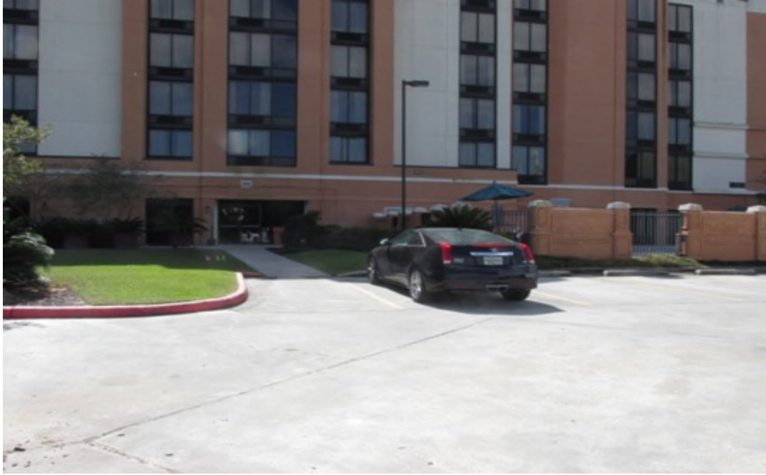
Existing pool and deck protrude far from building on north side limiting or stopping any new road access
