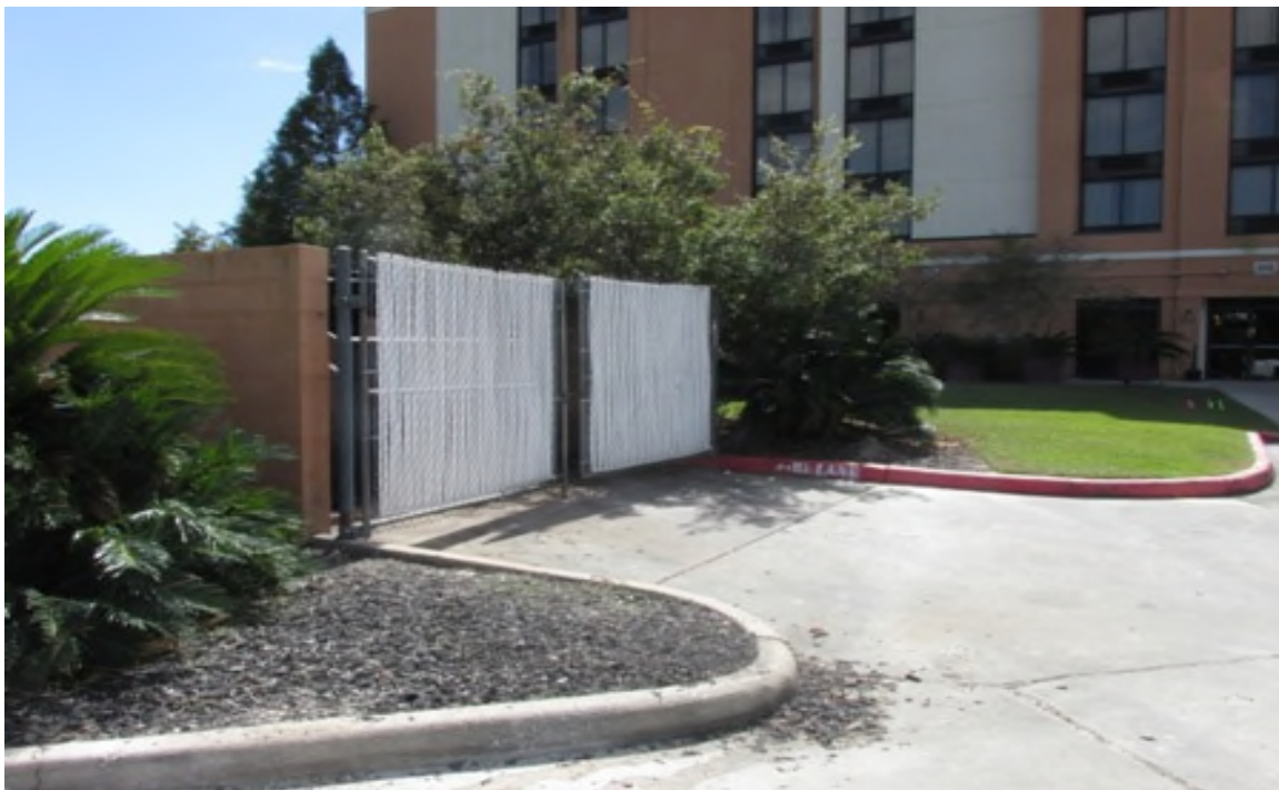
Narrow area between pool, deck and trash which overlaps fire lane
