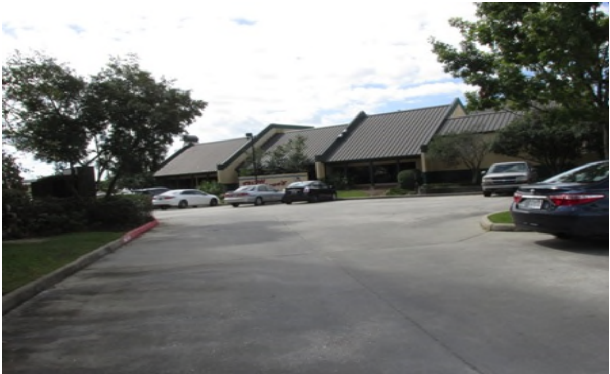
Ralph & Kacoo's east side, 4 feet or more below grade of hotel site along proposed Dijon Dr.
